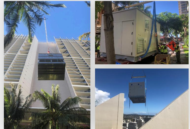
*Left: A cooling tower is lifted on the roof
